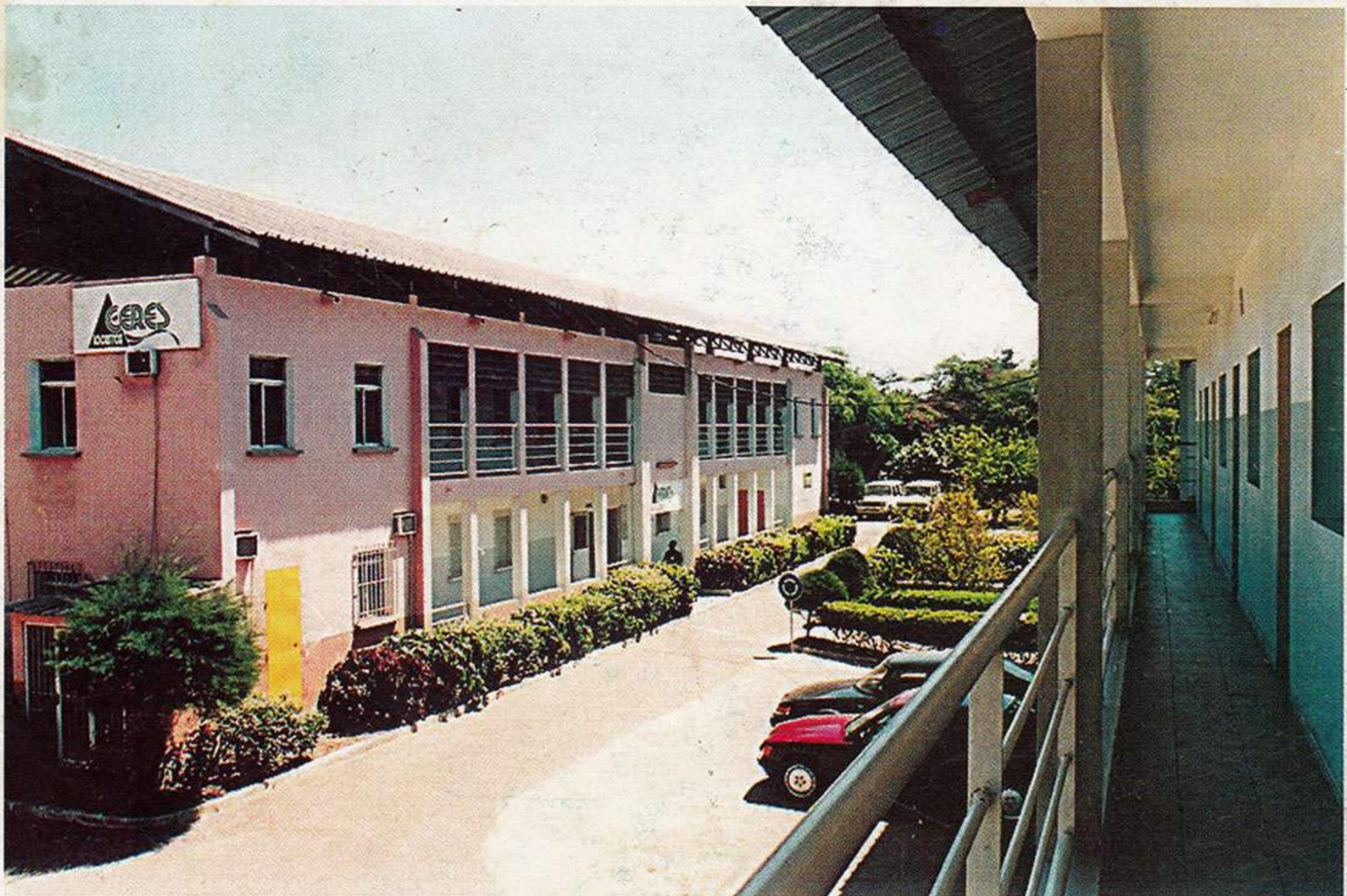
CERES LOCUSTOX Office and Laboratory Buildings - Km 15, Rte de Rufisque - Dakar Sénégal
